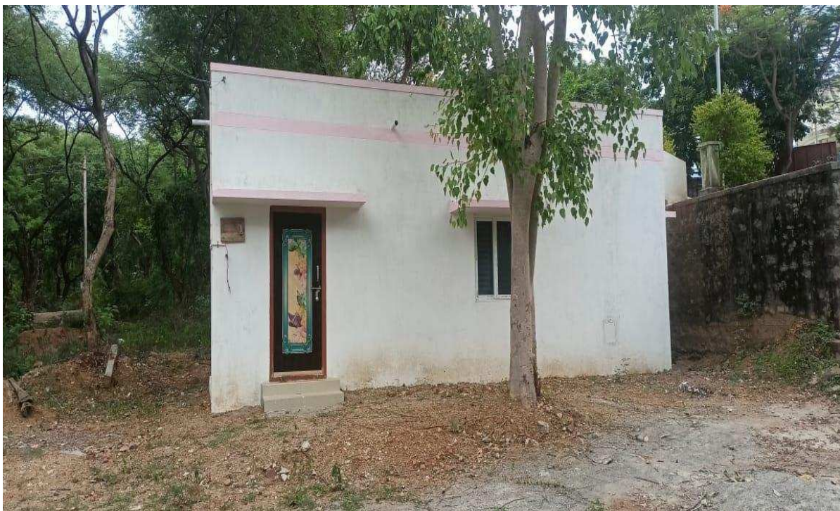
Retaining Room with Frontline Women Staff building in Theerthamalai Range - Newly Constructed
